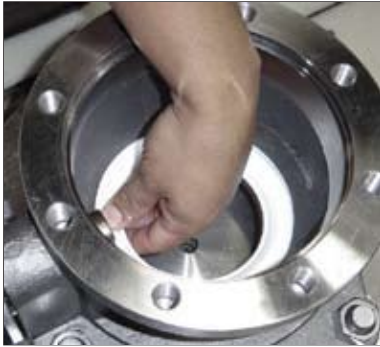
Figure 15 - Installing First Ball Seal
