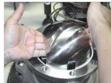
Figure 18 - Placing the Valve Ball
